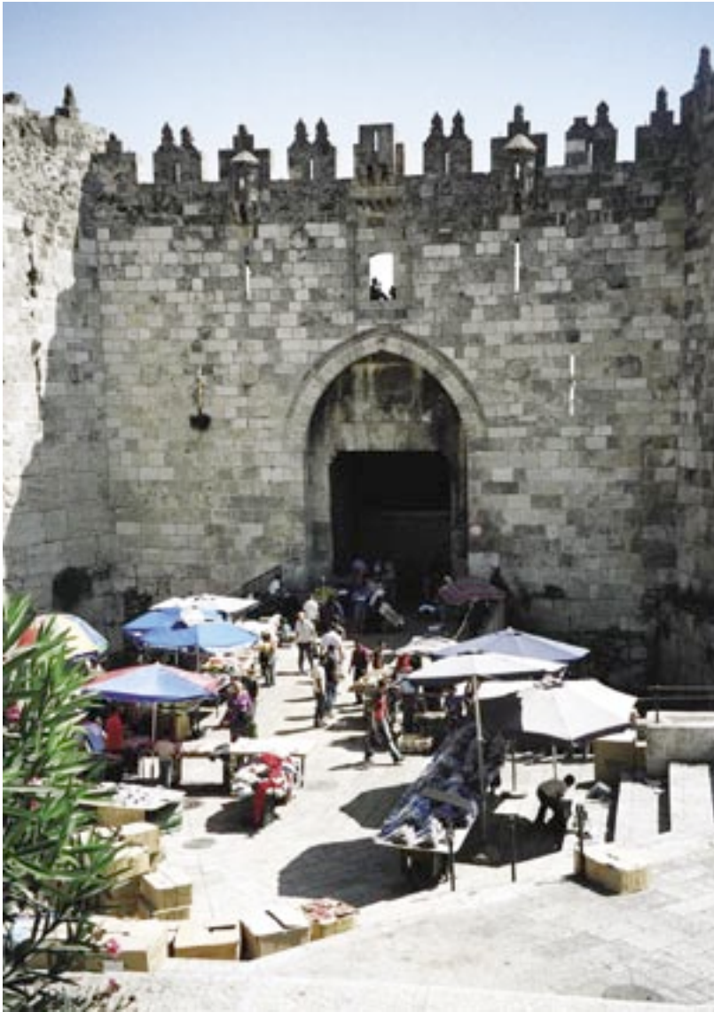
Figure 2: North side of Damascus Gate © Wendy Pullan
