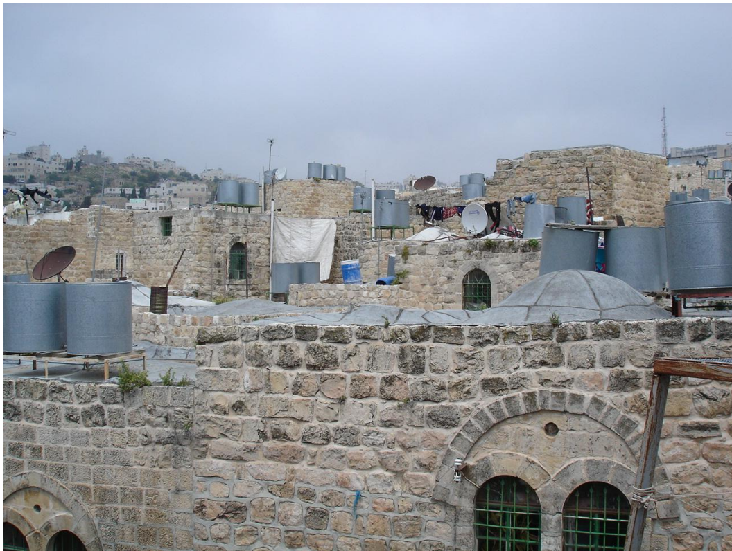
Figure 3: Old City's roofs (Photo courtesy Chiara De Cesari)
